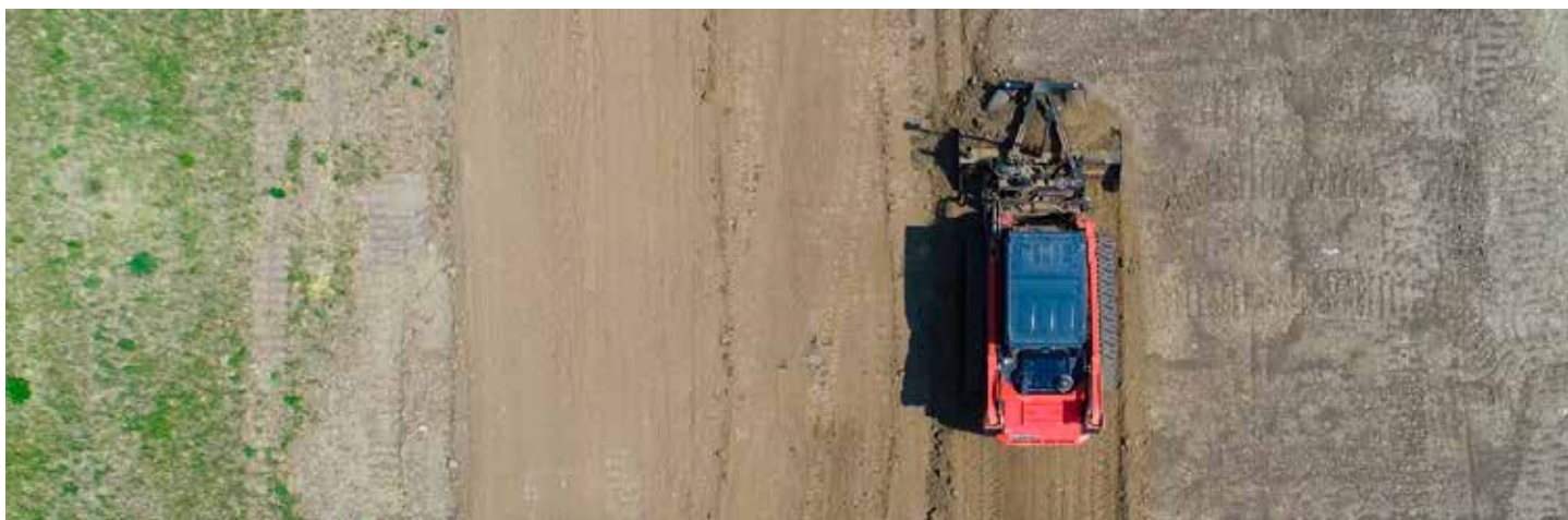
Operator John Shafer and the company's Kubota SVL97-2 are guided by Topcon's MC Mobile system in applying a 1% fall across a 250-foot-long garden plot area in the Berlin Farm subdivision in Delaware County, Ohio.
