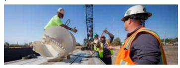
Goettle selected the 218 because it's a 110-ton crane rather than a 100-ton. "We got a little more oomph and it has a better chart than an H or an H2," Studt noted. "The extra 10 metric tons always helps, and it has a better reach."
