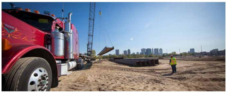
Under the Columbus skyline, Goettle Oiler Danny Smith awaits an incoming, 62-foot, 13,020-lb. beam. The beam will help form one of the Columbus site's 685 secant piles—a European technology that will provide support for the new, state-of-the-art facility.
