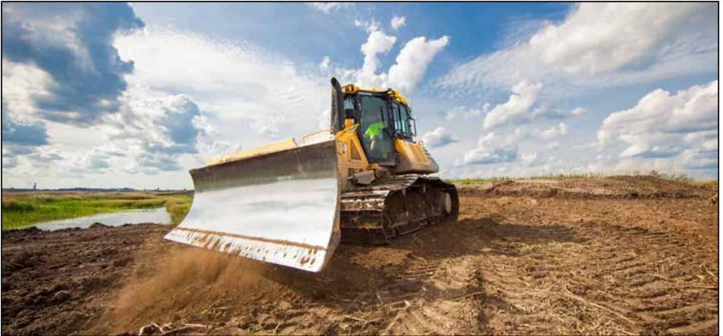
A Mark Haynes Construction Komatsu D61PXi performs site improvements at the Toledo Port Authority Confined Disposal Facility (CDF). Over 5 months, the iMC machine will help move over 500,000 cy of earth as the company clears the site, adds drainage structures and builds higher dikes.
